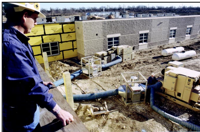
Figure 2: Construction drying equipment on a Texas job site.
