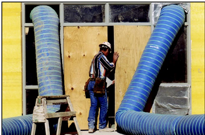
Figure 5: Temporary door to contain dry air.
