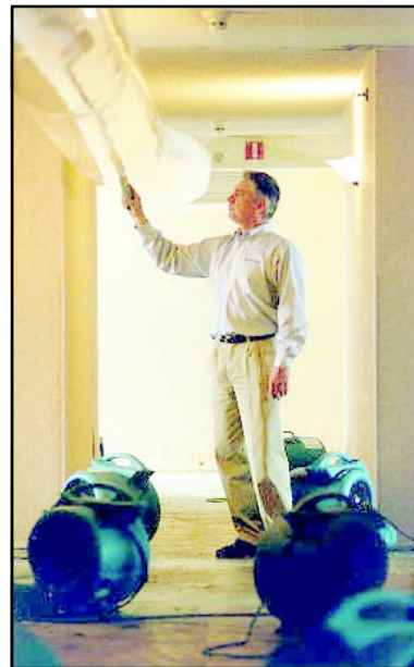
Figure 3 (left): Temporary dry air ductwork. Figure 4 (right): Air movers.
